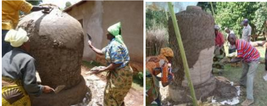
Farmers during construction of granaries
