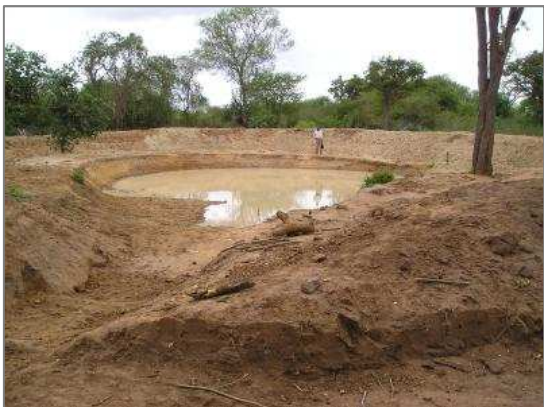
Fig. 15: Commonly found “Charco dam” for flood water diversion/runoff collection in Kenya ([InfonetBiovison, 2010])
